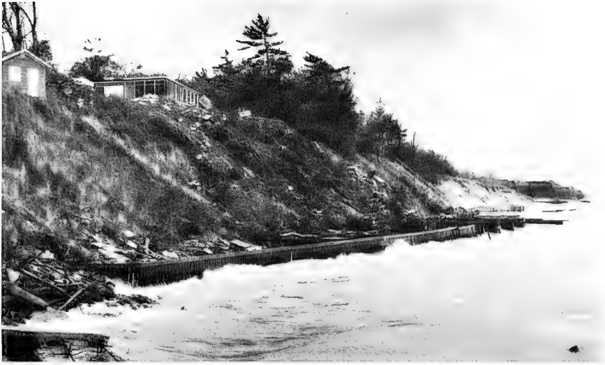
Figure 17. View of the downdrift cut from the southern end of the seawall. Heavy vegetation on the bluff slope indicates successful stabilization (16 October 1976).
